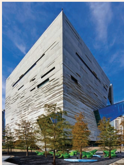
The exterior of the museum (left) consists of 700 unique precast panels. GPS technology was employed in the modeling of the lobby ceiling (right).
